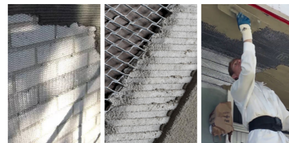
Brick wall reinforcement
